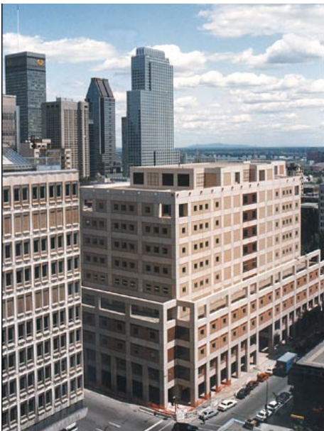
An external view of the The J.W. McConnell Building, just a stone's throw away from Parc du Mont-Royal, and home to the 2010 CASC annual conference.
